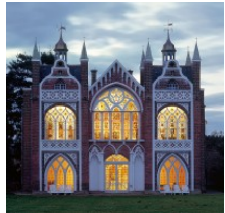
Fig. 1. The Gothic House, Wörlitz, Germany.
